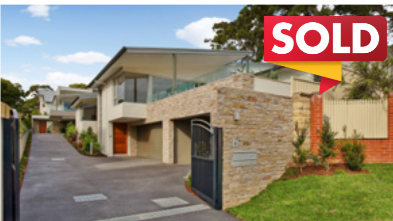
CARINGBAH SOUTH, Townhouse site
